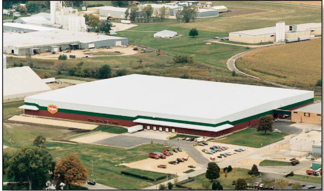
Butler executed three facilities of this size simultaneously—including projects in Wisconsin and Washington State—with local contracting support from the Butler Builder® Network. This plant-adjacent warehouse in Mendota, Illinois measures 239,850 sq. ft.
