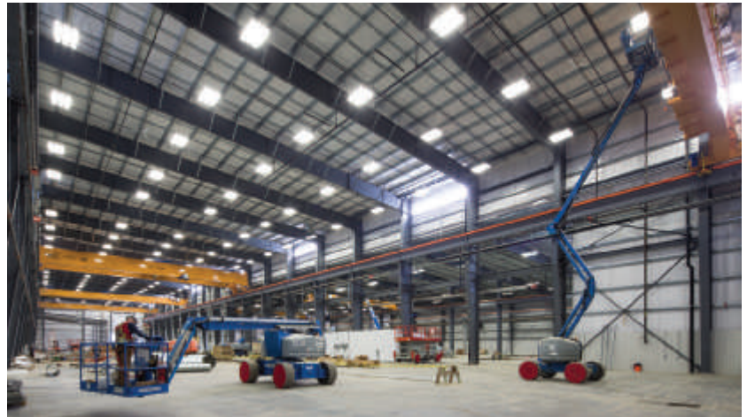
The facility includes several joined structures, with large spans and great heights to accommodate 40-foot crane hook needs.
